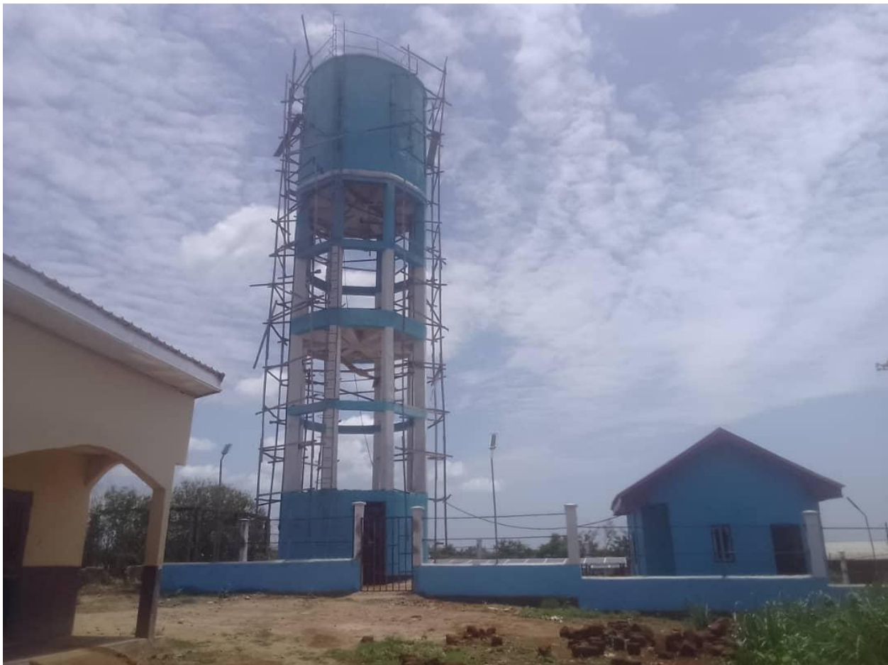
Image of newly installed borehole.
