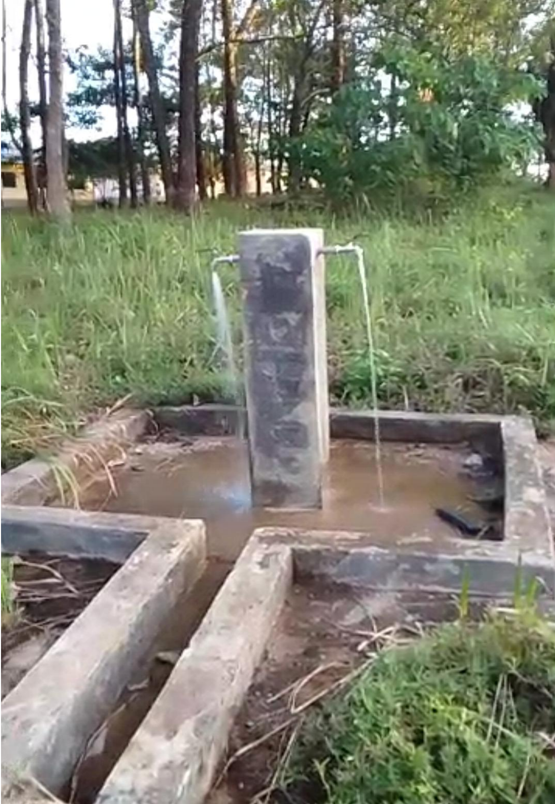
Installation of New Water Taps in Target Communities
